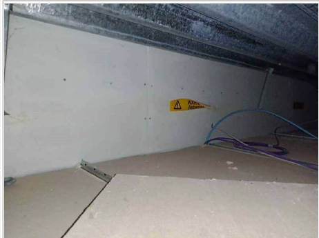
Photo No. 26 - Firebreak panels in ceiling void above door and surround leading to Art C 019 and associated debris
