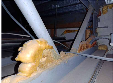
Photo No. 22 - Firebreak panels in ceiling void adjacent Office C004 (accessed via ceiling void in Art C 024) (as sample DG004868)
