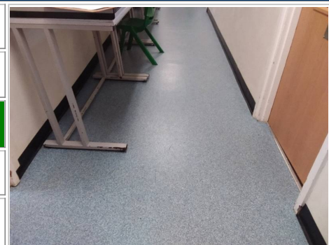
Photo No. 3 - Vinyl floor tiles (beige) and bitumen adhesive below (possibly below new floor covering)
