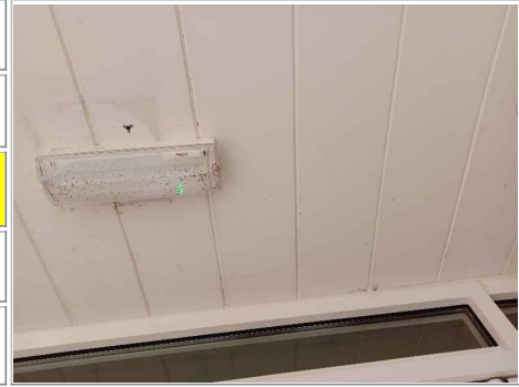
Photo No. 40 - Fixed ceiling panels to entrance porch to Circulation C 039 (small areas require remedial action)
