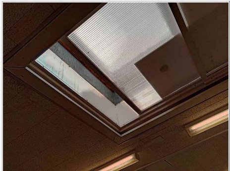
Photo No. 14 - Skylight cheeks to skylights (3 no.) continuing above sealed sliding windows (small areas require remedial action) (as sample DA005505)
