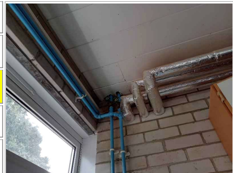
Photo No. 6 - Fixed ceiling panels (small areas require remedial action) (as sample DA005504)
