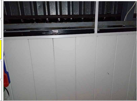
Photo No. 4 - Fixed ceiling panels to east side of room (small areas require remedial action) (as sample DA005504)
