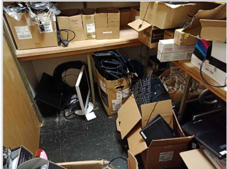
Photo No. 29 - Vinyl floor tiles (black) and bitumen adhesive below (small areas require remedial action) (as sample DA005518)
