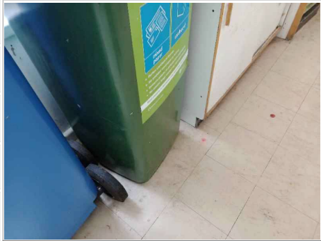
Photo No. 25 - Vinyl floor tiles (lighter cream) to centre of room and bitumen adhesive below
