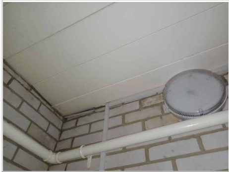
Photo No. 8 - Fixed ceiling panels (small areas require remedial action) (as sample DA005504)
