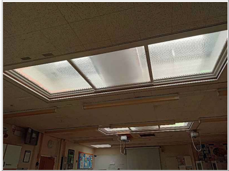
Photo No. 12 - Skylight cheeks to skylights (4 no.) continuing above sealed sliding windows (as sample DA005505)
