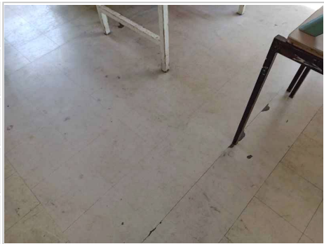
Photo No. 25 - Vinyl floor tiles (lighter cream) to centre of room and bitumen adhesive below
