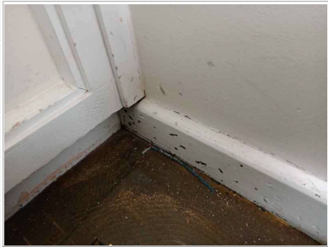
Photo No. 29 - Vinyl floor tiles (black) and bitumen adhesive below (small areas require remedial action) (as sample DA005518)
