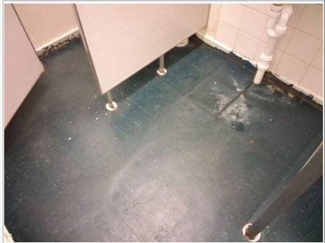
Photo No. 35 - Vinyl floor tiles (orange) and bitumen adhesive below (small areas require remedial action)
