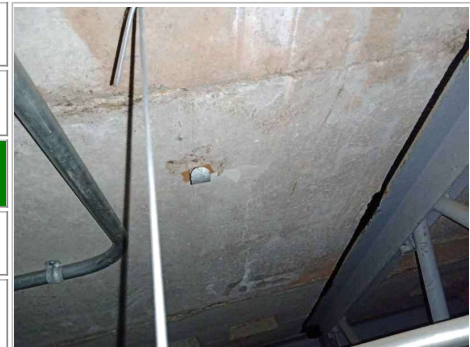
Photo No. 2 - Damp proof course above steel joists within ceiling void (as sample DA005536)
