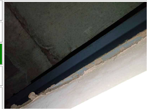
Photo No. 2 - Damp proof course above steel joists within ceiling void (as sample DA005536)
