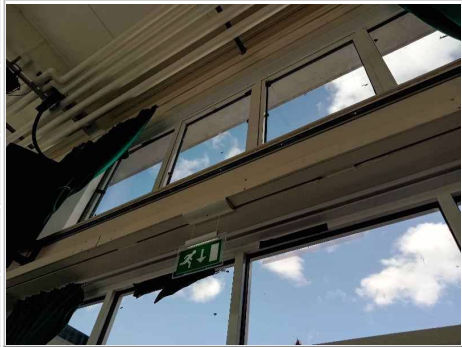
Photo No. 20 - Packing panels between metal conduit and wall at high level to east side of room
