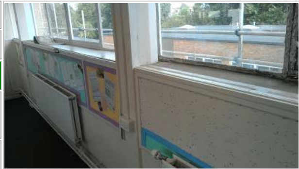
Photo No. 103 - Vinyl sheeting (grey) to window sills to south side of room (possibly below new PVC window sills)
