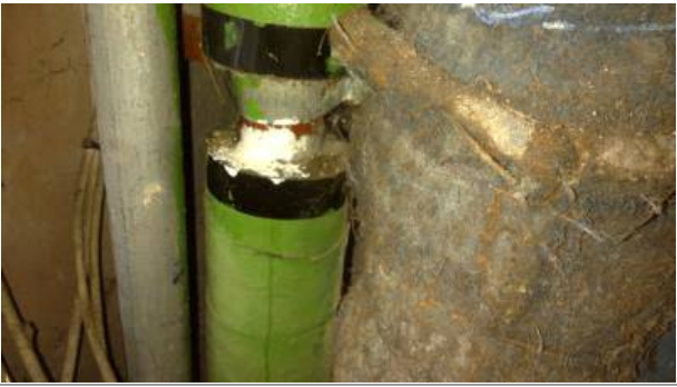
Photo No. 77 - Paper lining to pipework behind glassfibre insulation within riser to north side of room*
