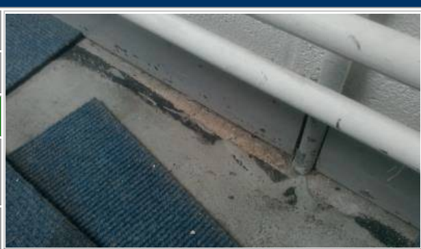
Photo No. 25 - Bitumen adhesive to floor continuing below screed below carpet (possibly below new floor covering)
