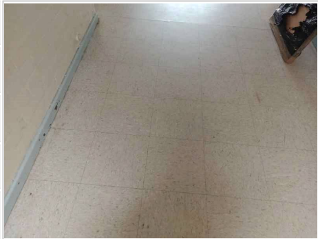
Photo No. 53 - Vinyl floor tiles (light grey) and bitumen adhesive below (as sample AQ001883)
