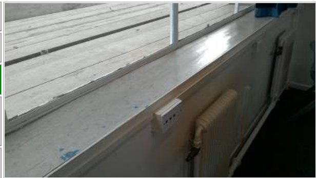
Photo No. 87 - Vinyl sheeting (grey) to window sills to south side of room (possibly below new PVC window sills) (as sample AQ001942)
