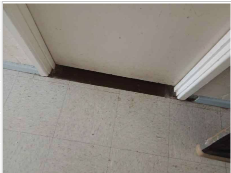
Photo No. 54 - Vinyl floor tiles (brown) adjacent door thresholds to north side of room and bitumen adhesive below
