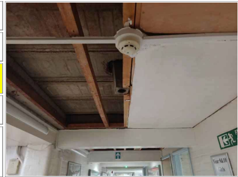
Photo No. 29 - Residue around nail holes outside Store A 057 and W.C. A 055 to wooden ceiling joists behind plyboard paneling (approx 10-12m2)
