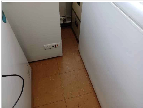
Photo No. 23 - Vinyl floor tiles (beige) to floor and side of window sill and bitumen adhesive below
