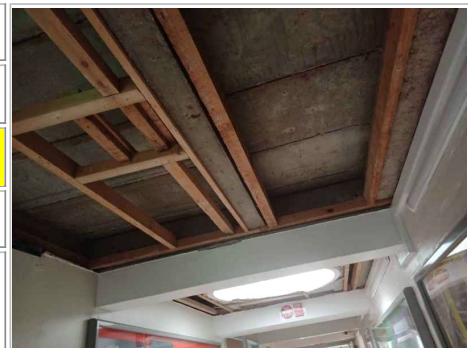
Photo No. 31 - Residue to timber frame work to ceiling adjacent A 056 and A058 area (sealed behind plyboard)
