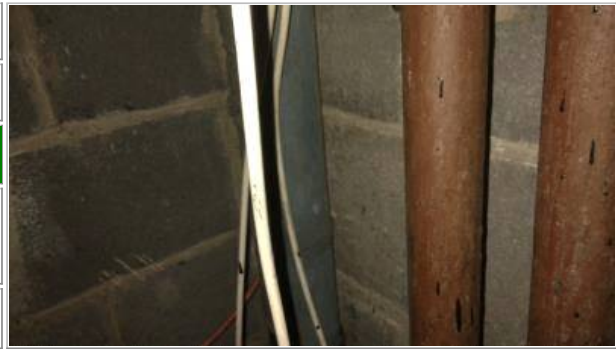
Photo No. 96 - Paper lining to pipework below glassfibre insulation within riser in southwest corner of room* (as sample AG001058)
