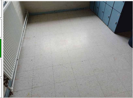
Photo No. 44 - Vinyl floor tiles (light grey) and bitumen adhesive below (as sample AQ001883)
