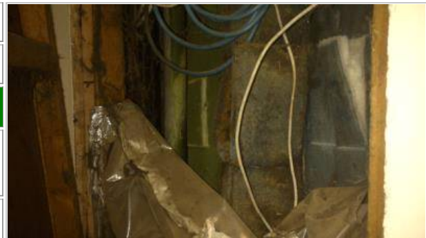
Photo No. 15 - Paper lining to pipework behind glassfibre insulation within riser to northeast side of room adjacent door to Learning Resource Centre A 014* (as sample AG001050)
