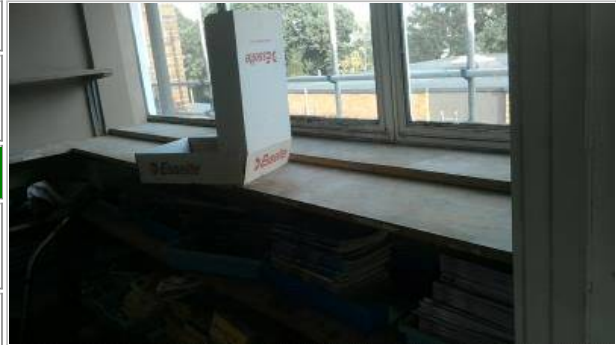
Photo No. 100 - Vinyl sheeting (grey) to window sill and bitumen adhesive below (possibly below new PVC window sills) (as sample AQ001900)
