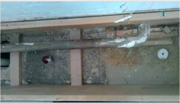
Photo No. 88 - Vinyl floor tiles (grey) below carpet adjacent pillar and adhesive below (possibly below new floor covering)
