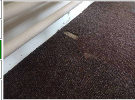
Photo No. 101 - Vinyl floor tiles (grey) below carpet and modern screed and bitumen adhesive below
