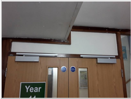
Photo No. 78 - Infill panels behind timber panelling above doors leading to Circulation B106 (as sample DG004861)
