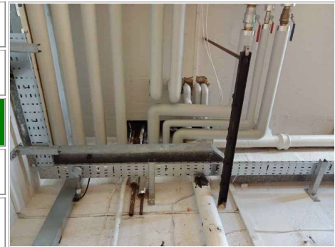
Photo No. 3 - Paper lining to pipework below glassfibre insulation within riser in ceiling in southwest corner of room (as sample AG001050)
