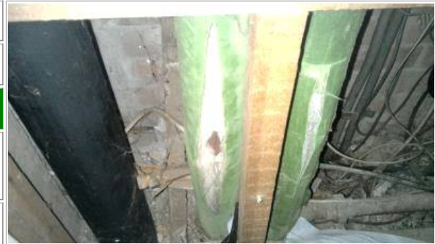
Photo No. 13 - Paper lining to pipework below glassfibre insulation within riser in southwest corner of room
