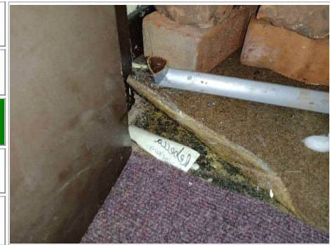
Photo No. 3 - Paper lining to pipework below glassfibre insulation within riser in ceiling in southwest corner of room (as sample AG001050)
