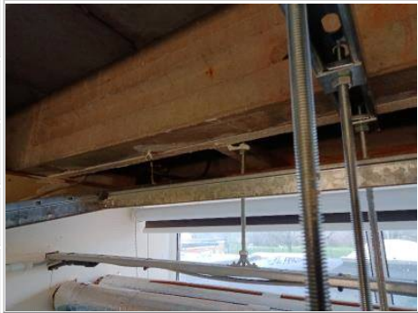
Photo No. 36 - Residue to timber frame above pipework to west area above suspended ceiling tiles
