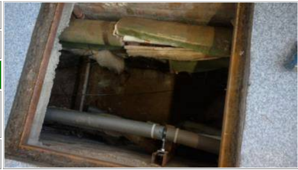
Photo No. 16 - Paper lining to pipework behind glassfibre insulation within floor duct to east side of room (inspected floor duct from hatch only)* (as sample AG001050)
