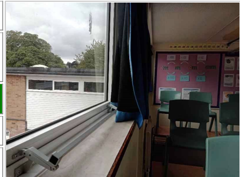
Photo No. 74 - Vinyl sheeting (grey) to window sills to south side of room and bitumen adhesive below (as sample AQ001900)
