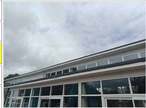
Photo No. 114 - Soffit boards to perimeter of Dining Hall A 025, Stage A 035 and Sports Hall A 037 (paint peeling throughout) (as sample AM000165 )
