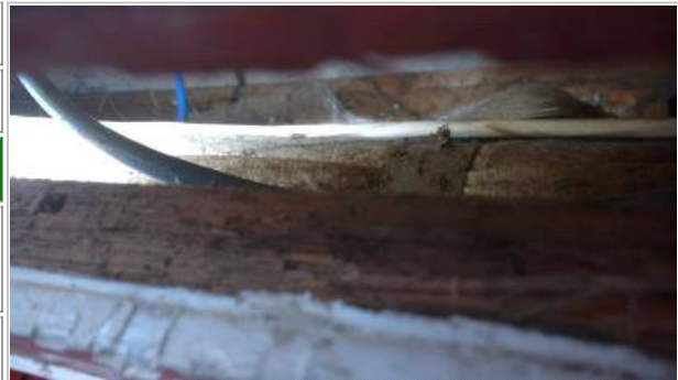
Photo No. 110 - Paper lining to pipework behind glassfibre insulation behind boxing to west side of building adjacent Caretaker's Office A 069* (as sample AG001050)
