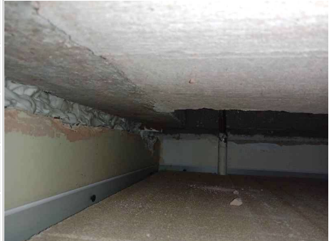
Photo No. 39 - Panel residue to surfaces / areas at top of solid wall to south side of room and to top of cylindrical metal conduit housing cables above suspended ceiling grid (residue is surface sealed with silicone at top of wall and with multi-purpose filler on the conduit)
