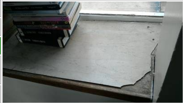
Photo No. 87 - Vinyl sheeting (grey) to window sills to south side of room (possibly below new PVC window sills) (as sample AQ001942)
