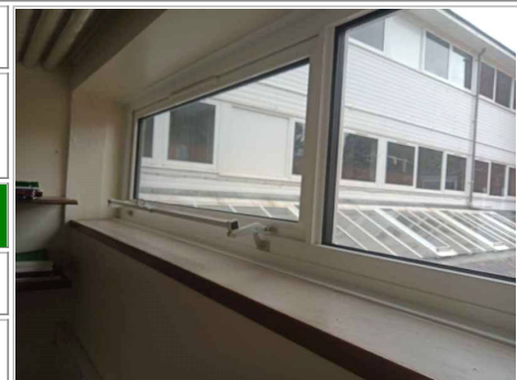
Photo No. 83 - Vinyl sheeting (grey) to window sill to east side of room and bitumen adhesive below (as sample AQ001900)
