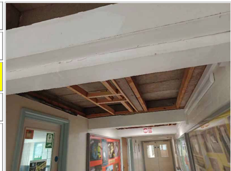
Photo No. 30 - Residue around nail holes outside Office A 056 to wooden ceiling joists behind plyboard paneling (approx 10-12m2)
