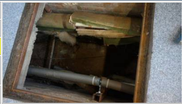
Photo No. 17 - Paper lining debris within floor duct to east side of room (inspected floor duct from hatch only)* (as sample AG001050)
