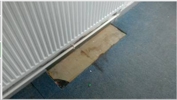
Photo No. 24 - Vinyl floor tiles (green) to northwest area of room and bitumen adhesive below (possibly below new floor covering)
